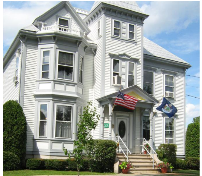
Kennebec Behavioral Health's Winthrop Clinic is familiar building on Old Lewiston Road.
